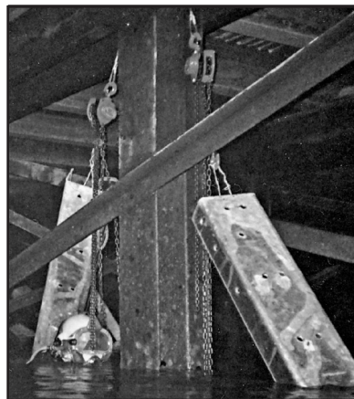
Steel pile reinforcement dock repair.
