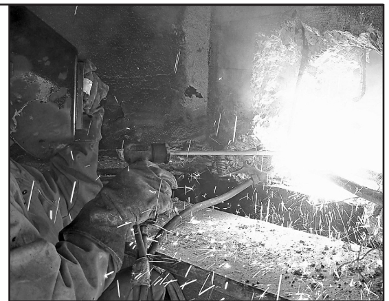
Cutting a rebar at Beesleys Point Bridge.
