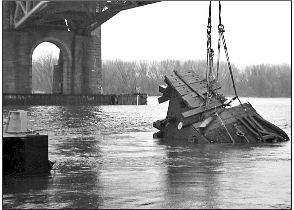
Hydro-Marine's handiwork includes the dismantling of a damaged fender timber system under the Tacony-Palmyra Bridge.
