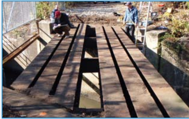
Roebling Bridge at the project start.
