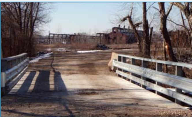
Roebling Bridge at project completion.
