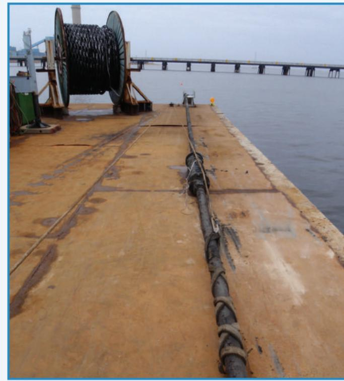
attach the slings/rigging. Cranes were then used to pull the underwater cable to the surface and anchor it onto the barge. What made this process even more difficult was the severe winter weather, as most faults usually occur in late fall or early spring, not in the dead of winter.
